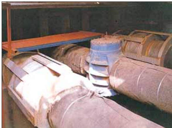
Fig. 42. Pressure balanced expansion joint
