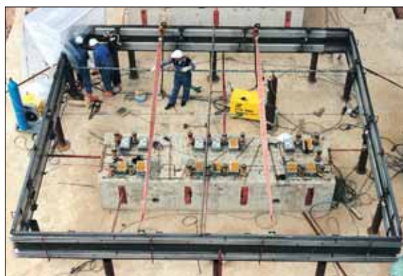
Fig. 25. Mounting of rectangular expansion joint
